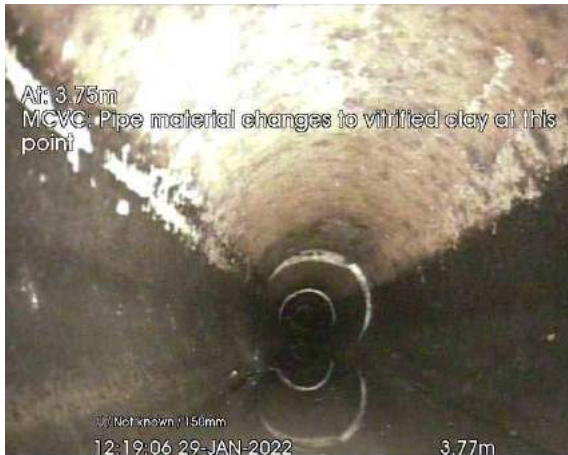
MH2 TO MH1_3-77m_121906.jpg, 00:00:24, 3.77 m Pipe material changes to vitrified clay at this point
