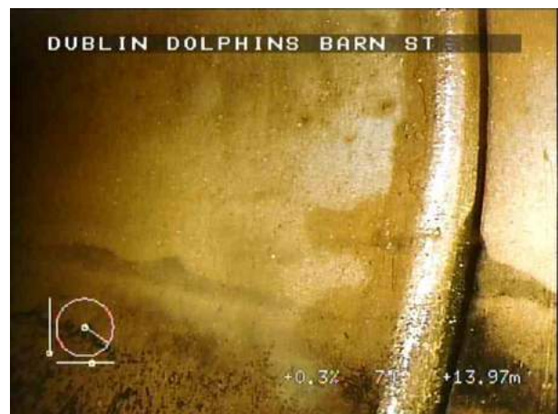
SMH4X_f82a13ab-69c4-45fd-8f68-8b0b8f6aada8_20220408_125015_918.jpg, 00:02:34, 13.97 m Open joint, medium
