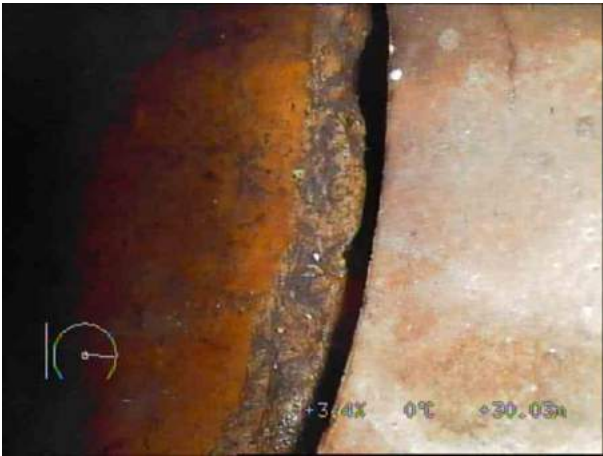
SMH3X_0aac7fce-5a23-446e-884d-486e70784976_20220408_103502_848.jpg, 00:13:00, 30.03 m Open joint, large
