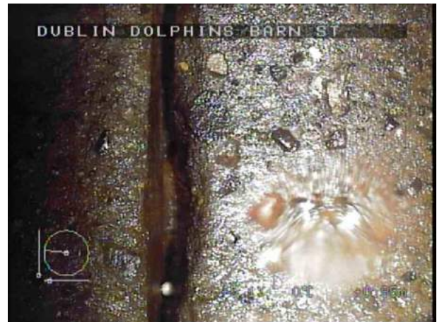
SMH2X_0889b6b3-45e6-4b41-bbfa-a42acf304ac4_20220408_100034_943.jpg, 00:00:27, 0.85 m Open joint, medium
