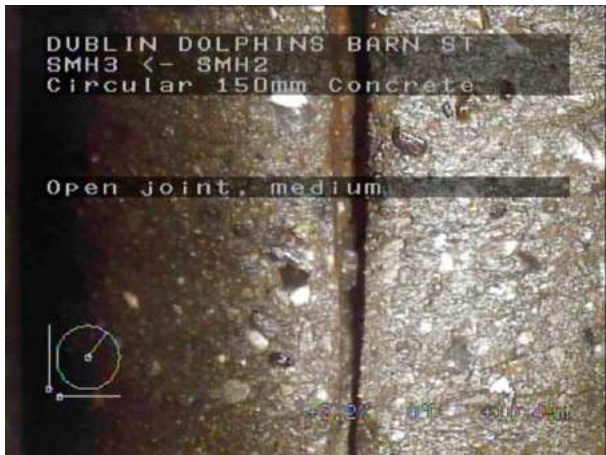
SMH3X_ee8eff8b-ef12-4309-8494-48da32b7e79d_20220408_101528_559.jpg, 00:03:34, 10.49 m Open joint, medium
