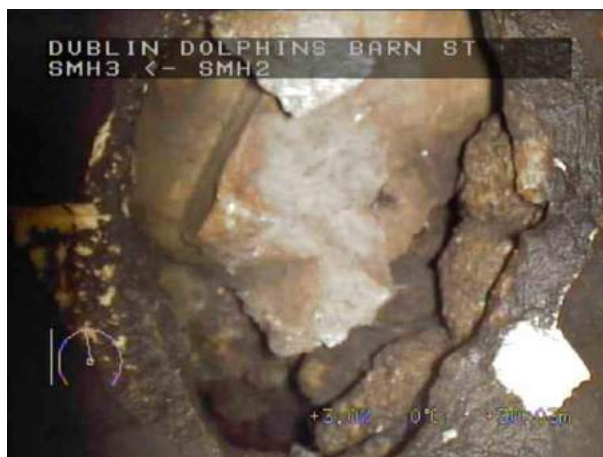
SMH3X_31bada83-1254-45d7-9f25-eaef24bba3c3_20220408_103439_621.jpg, 00:12:44, 30.03 m Hole in drain or sewer from 11 o'clock to 1 o'clock
