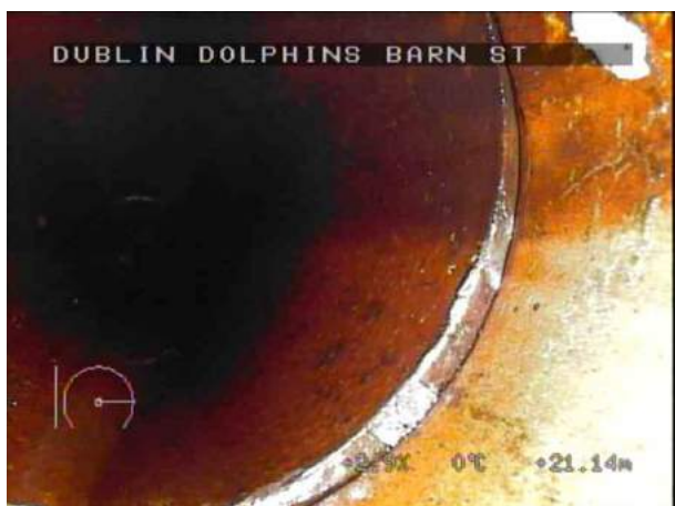
SMH3X_b2ac8f39-db7c-4314-b07c-01876c25bebb_20220408_102842_873.jpg, 00:08:54, 21.14 m Joint displaced, large
