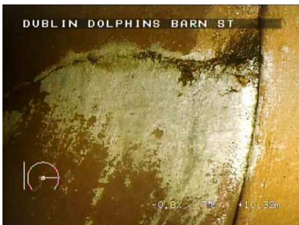
SMH4X_9f0fee19-06ee-4eac-a4d9-c5c9cc5831d0_20220408_124933_278.jpg, 00:01:58, 10.32 m Fractures, radiating from 3 o'clock to 4 o'clock
