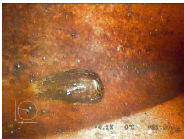
SMH3X_d48bc823-7a6c-4735-a61d-b64428dd3433_20220408_102923_372.jpg, 00:09:18, 21.20 m Deformed sewer or drain, 5%
