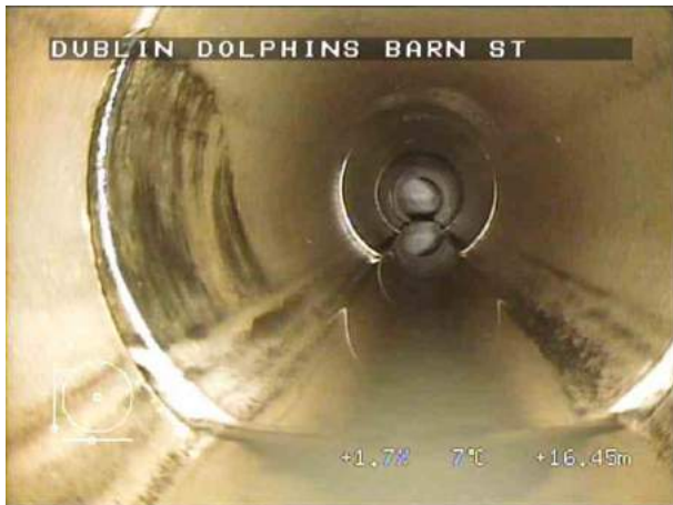
SMH4X_640e99a1-0852-4f0b-bc90-f30d2a366878_20220408_125041_365.jpg, 00:02:54, 16.45 m Joint displaced, large
