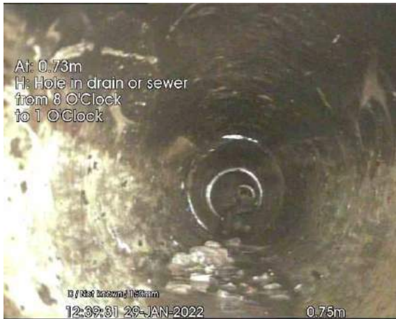
MH1 TO MH2_0-75m_123931.jpg, 00:00:09, 0.75 m Hole in drain or sewer from 8 o'clock to 1 o'clock
