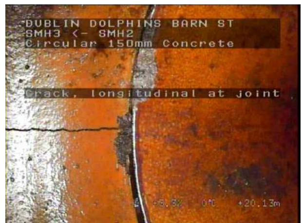
SMH3X_0ac6157f-b4ab-4ad9-8172-19cf6c224f8e_20220408_102755_481.jpg, 00:08:26, 20.13 m Crack, longitudinal at joint at 12 o'clock
