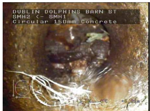
SMH2X_d3a5553c-1358-44da-8de2-f74cbf6eea60_20220408_100312_296.jpg, 00:02:22, 6.01 m Junction at 9 o'clock, 100mm dia
