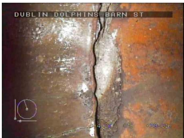
SMH3X_e097369b-9d07-4f80-b9f6-642262c70cb6_20220408_103357_091.jpg, 00:12:25, 29.61 m Open joint, large
