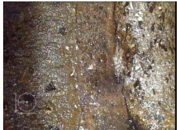
SMH3X_f949510e-b4f6-4394-8afe-2daf860bfc1d_20220408_101348_771.jpg, 00:02:23, 8.52 m Open joint, large
