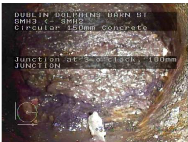
SMH3X_a0c2e369-32cc-4cbc-b45b-fe9c2527e042_20220408_101438_189.jpg, 00:02:50, 9.12 m Junction at 3 o'clock, 100mm dia, OLD JUNCTION
