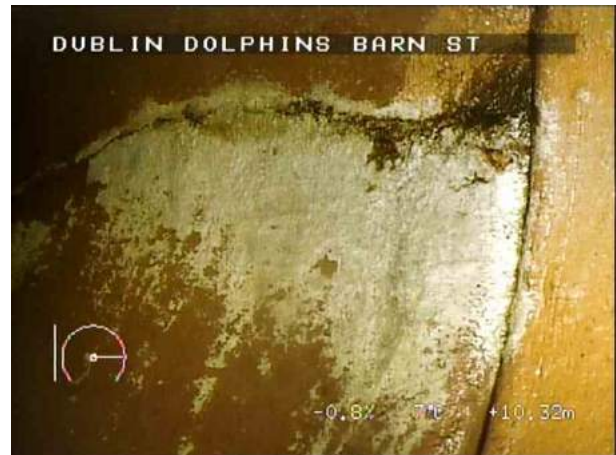
SMH4X_92a2a218-7c0a-4af8-a8bc-a1bf08f2b202_20220408_124933_070.jpg, 00:01:58, 10.32 m Fractures, radiating from 3 o'clock to 4 o'clock
