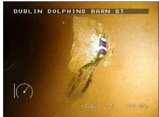
SMH4X_81fbdfc0-ff1d-458a-a526-edb992863217_20220408_125119_158.jpg, 00:03:20, 19.60 m Hole in drain or sewer from 1 o'clock to 2 o'clock
