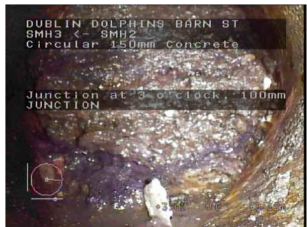
SMH3X_97c281b6-352d-4a2b-aacf-9862c78501cb_20220408_101439_675.jpg, 00:02:50, 9.12 m Junction at 3 o'clock, 100mm dia, OLD JUNCTION
