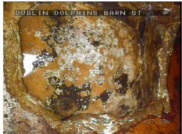
SMH3X_4bc7a12c-afa4-49e1-a5d1-6b8698e8d898_20220408_102308_252.jpg, 00:06:54, 17.63 m Deformed sewer or drain, 10%, OLD CONNECTION
