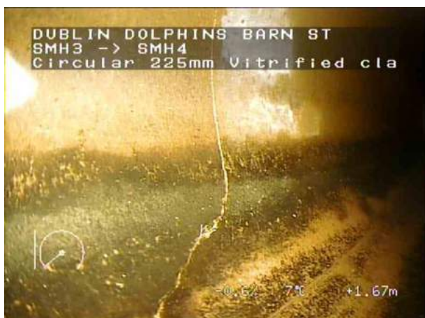
SMH3X_5d898e02-e1ea-4f7e-bf14-5680b51cd7bd_20220408_124241_795.jpg, 00:00:49, 1.67 m Cracks, radiating from 8 o'clock to 10 o'clock
