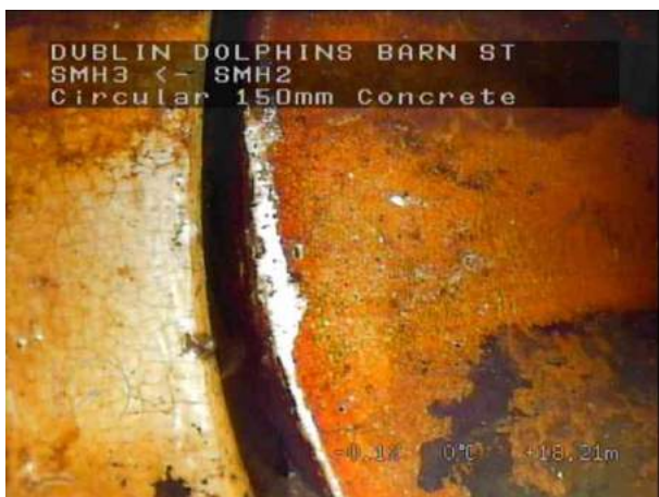
SMH3X_4560511f-a8a0-4761-b103-2ad8f21897b7_20220408_102426_372.jpg, 00:07:51, 18.21 m Open joint, medium
