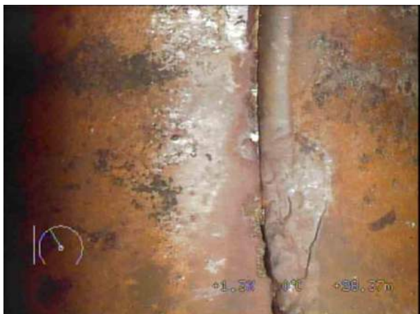
SMH3X_2d4f37a4-ef05-4947-9a4c-4fce43f26fed_20220408_103232_340.jpg, 00:11:25, 28.37 m Deformed sewer or drain, 10%
