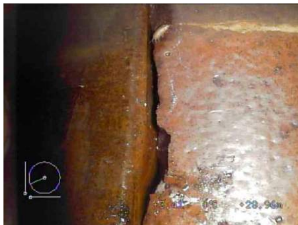
SMH3X_c4e3b749-1326-407f-856d-6befd816f5e4_20220408_103324_828.jpg, 00:12:01, 28.96 m Open joint, large
