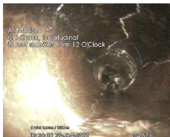
MH2 TO MH1_54-87m_122630.jpg, 00:05:14, 54.87 m Crack, longitudinal, in roof slab at 12 o'clock
