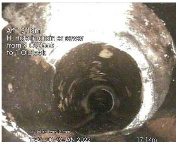
MH2 TO MH1_17-14m_122100.jpg, 00:01:56, 17.14 m Hole in drain or sewer from 9 o'clock to 1 o'clock
