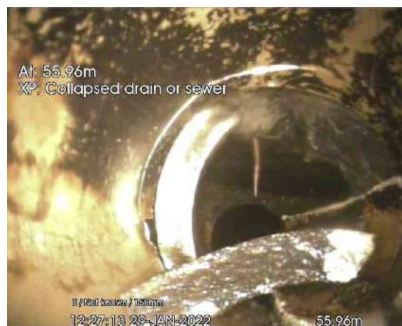
MH2 TO MH1_55-96m_122713.jpg, 00:05:34, 55.96 m Collapsed drain or sewer
